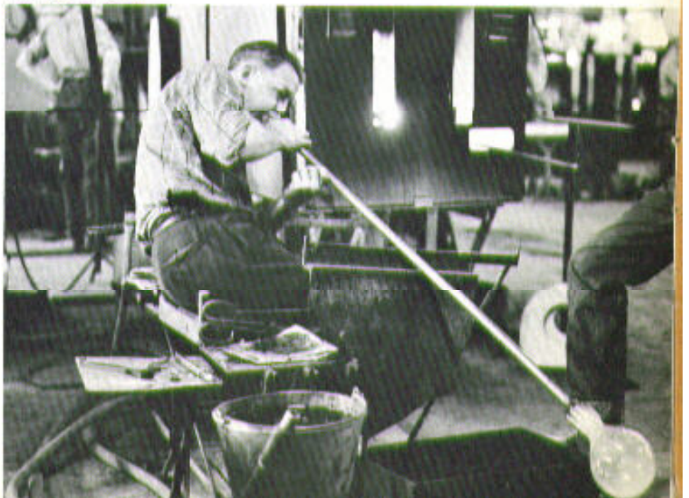
The glass is blown
